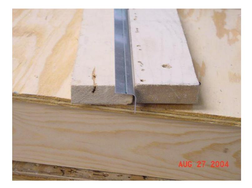
Notice above how you set the stiffener in between two boards in order to back-drill through the outside of the pre-punched skin.
