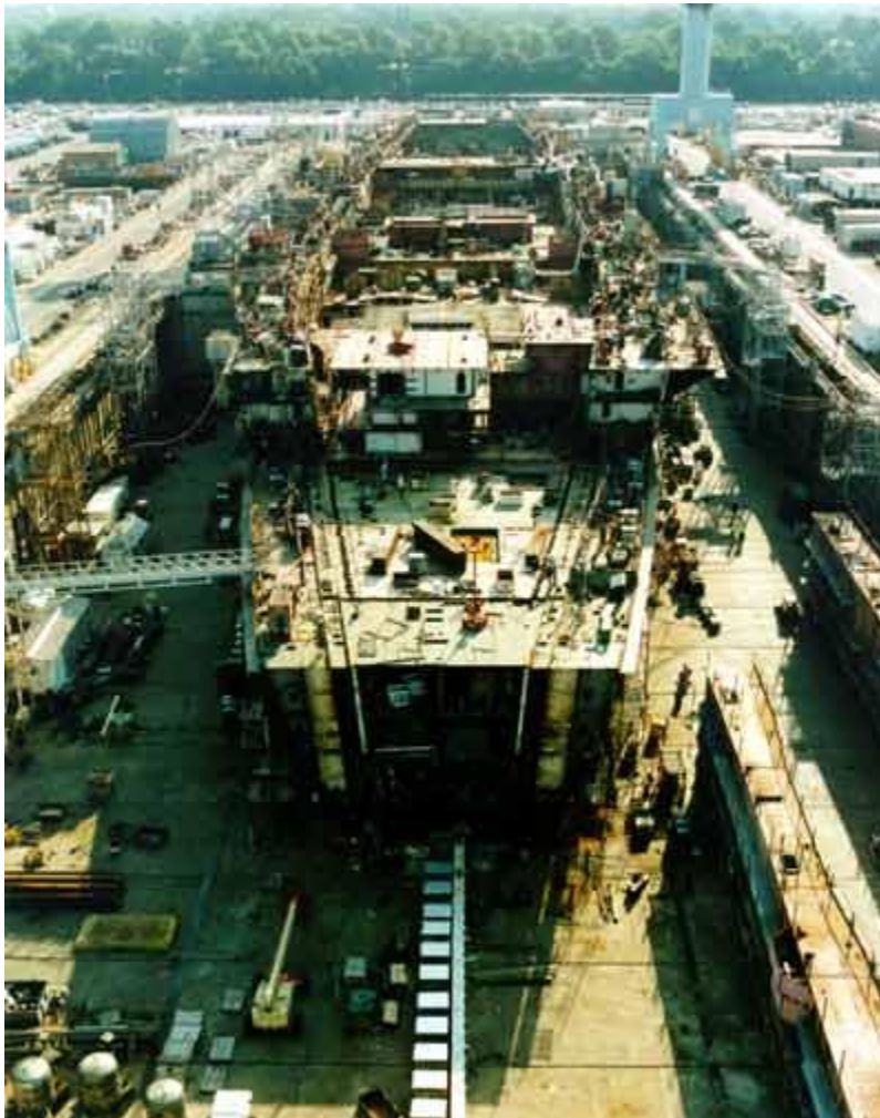
Photo courtesy Northrop Grumman Newport News The USS Ronald Reagan, under construction in the Northrop Grumman Newport News dry dock
