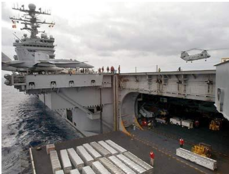
Photo courtesy U.S Navy One of the hydraulic elevators on the USS George Washington, lowered to the hangar deck
