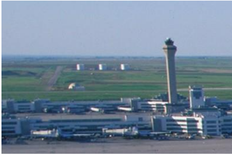
Photos courtesy Denver International Airport View of Denver International Airport showing the three fuel islands in the background
