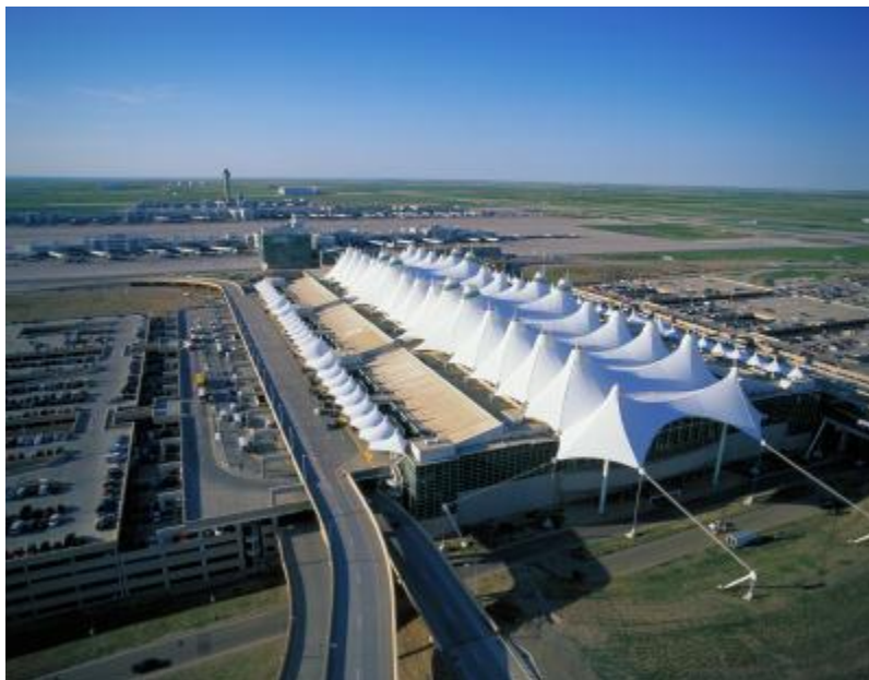
Photo courtesy Denver International Airport Jeppesen Terminal (middle), showing access road, passenger drop-off/pick-up areas (left) and parking garages (right)
