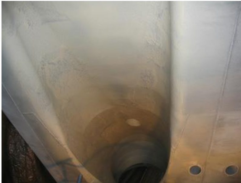
Photo courtesy U.S. Navy Waterjet tunnel under construction
