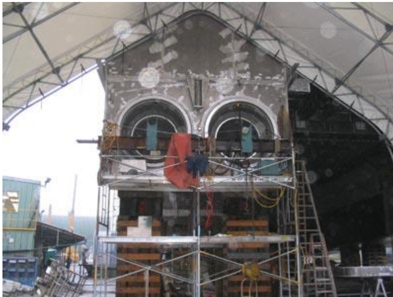
Photo courtesy U.S. Navy Housing for two of the four waterjets under construction
