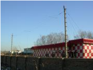
The NDB station co-located with Middle Marker of Beijing Capital International Airport ILS RWY36L
