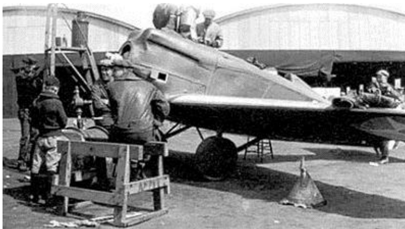
Mechanics at work on the Verville-Sperry Racer
