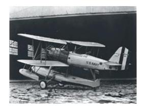
**O2U-3** an O2U-2 with revised wing rigging, redesigned tail surfaces and R-1340-C engine; 80 were built.
