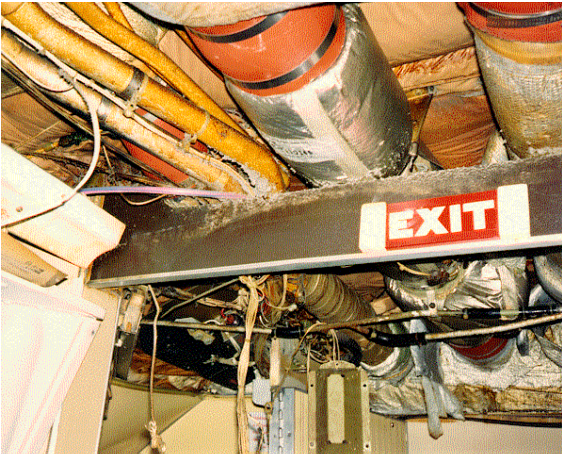
FIGURE 3-7. CROWN AREA INSPECTION
