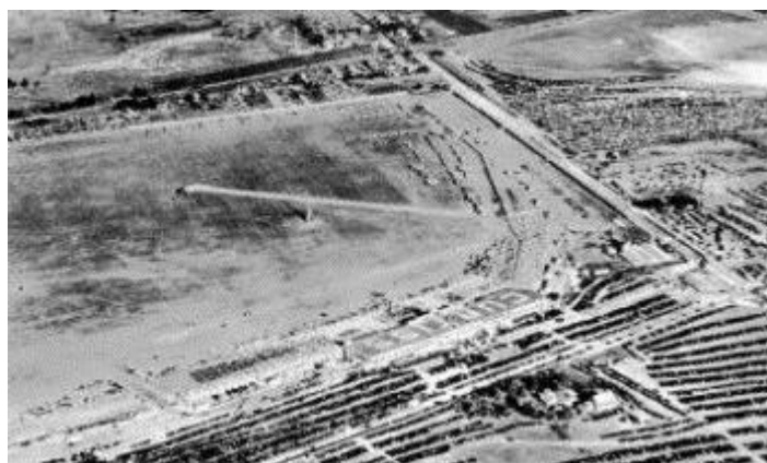
Aerial view of the Air Race site at Curtiss Field
