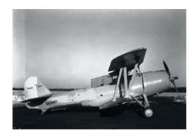
One two-place biplane was built for the Navy and first flight was in 1936. It was basically a SBU-2 with retractable landing gear. It was offered to the Navy at the same time as XSB2U-1 in case the monoplane was not bought by the Navy
