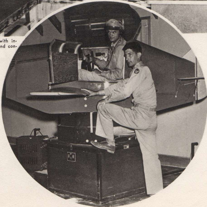
Link trainer—the plane that flies without leaving the classroom floor.
