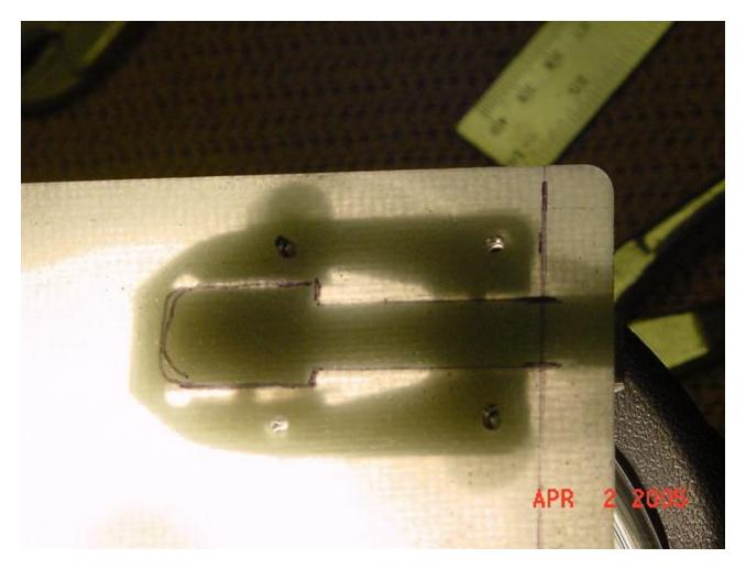
I sat the Hartwell latch on the bottom of the oil door and hit the back with a light. That made a nice silhouette, and I used a sharpie to trace the outline of the latch. Then I used drilled, files and a coping saw blade to cut out the recess for the latch in the oil door. It takes a lot of fine work to even get the recesses decent. I went back and hit it all with sandpaper afterwards so that when I operate the latch, the fiberglass edges aren't sharp around the latches.
