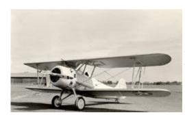
Only one XO4U-2 was built for the Navy to replace the XO4U-1, and its first flight was in 1932. The plane had metal wings with fabric covering and a metal monocoque fuselage. Records show delivery to the Navy but there are no records as to what use the Navy made of this airplane. It is assumed that it was used to evaluate the metal airframe structure.
